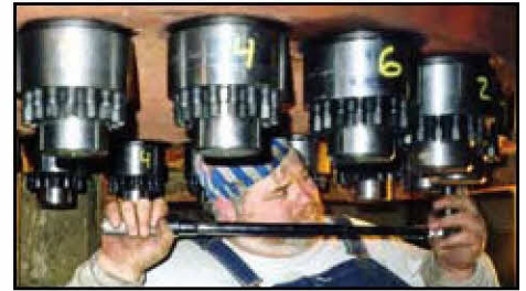
High pressure feedwater heater.
