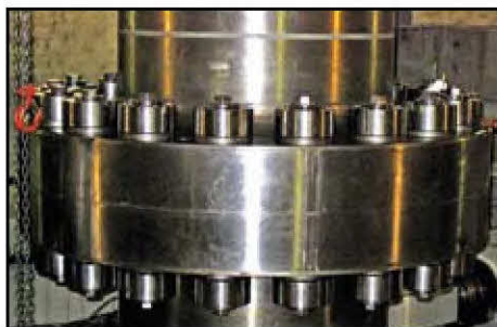
Coupling bolt installation utilizing Expansion Bolts.
