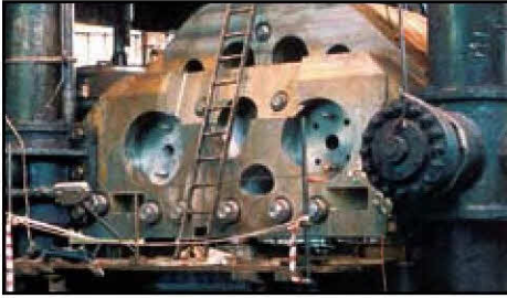
Press Platen repaired with tie bolts and Supernuts®.
