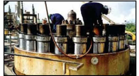
Large methanol reactor with 11" studs. Six hours with Superbolt® vs. two days with Hydraulic Tensioners.
