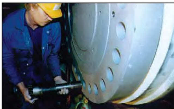
1200 MW Hydro Plant Nozzles on Pelton Turbines. Engineers were able to decrease the size of the nozzles with close spacing of the torquebolts®. Shown is the test plate being installed for hydro testing. Each 400 MW unit has five nozzles.
