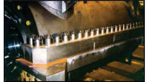
52 two inch tensioners on a centrifugal compressor were tightened in 2-1/2 hours.
