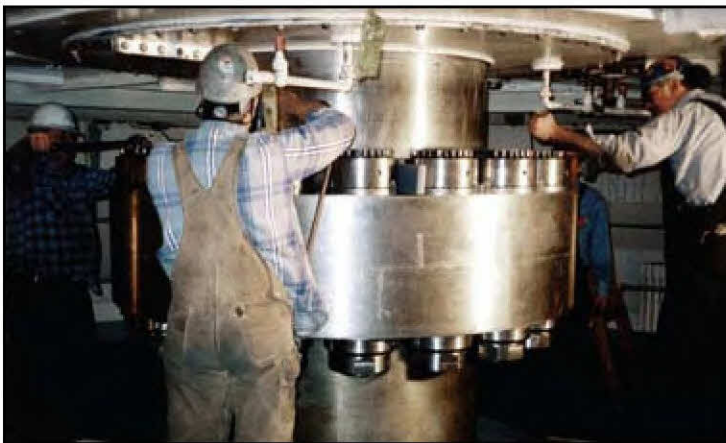
Kaplan turbine coupling, (18) 6-3/16" studs. The previous method required 150-250 man hours utilizing a 150 lb. "dead man", a 50 ton hydraulic ram, and a 250 lb. wrench. Supernuts® were installed in 2-1/2 hours using 1/2" air impacts and hand torque wrenches.
