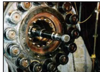
Ingersoll Rand boiler feed pump with 6" diameter studs (H650TX-600-8W). With air tools, tightening required only 2-1/2 hours.
